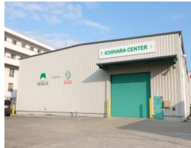
ecom LINCLE ICHIHARA Center (classified documents disposing facility)
