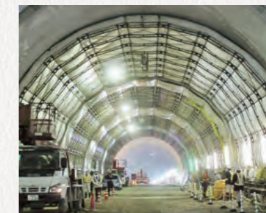
Construction site where Curemeister was used
