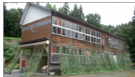
▼ The shuttered Azamihira Elementary School building.
